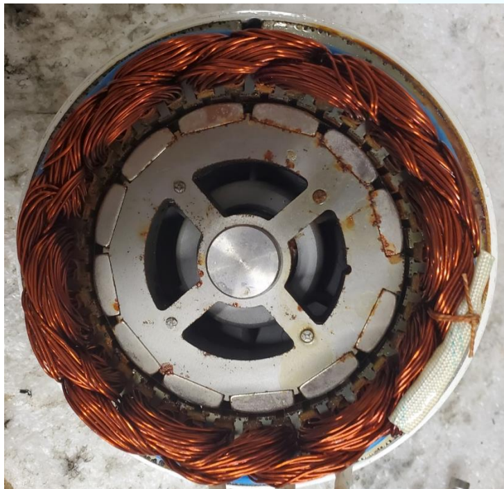
Photo 3 – Water infiltration – Customer photo
